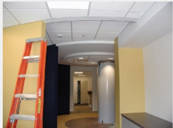
The nearly finished ITXC space, complete with rounded walls and ceilings
