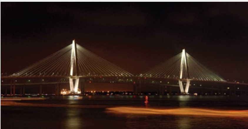
Grant Contracting installed the lighting, traffic controls, and signs for the new Arthur Ravenel Bridge. Opened in July 2005, the bridge spans Charleston’s Cooper River. (Photo courtesy of SCDOT)
