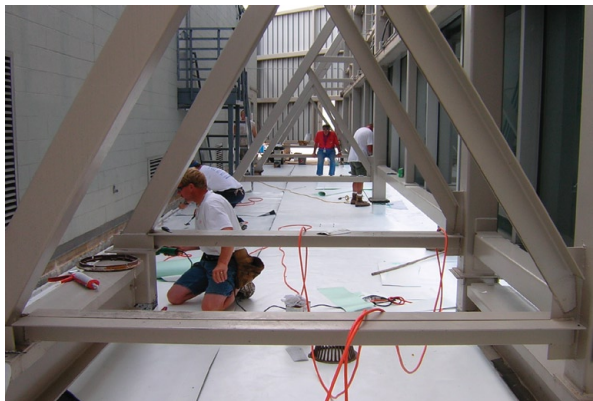
Belcher roofers at work on a commercial roofing project
