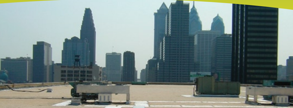
Philadelphia's skyline as seen from a newly-completed roofing project
